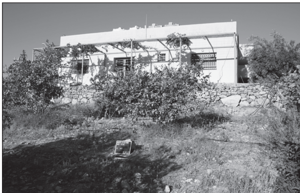
32. Site WS-026, remains of destroyed site (photo: A. Ahrens).
