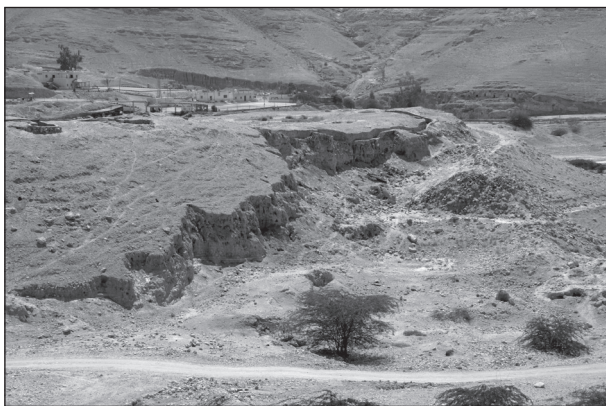
3. Collapsed northern flank of Tall Bulaybil (photo: A. Ahrens).
